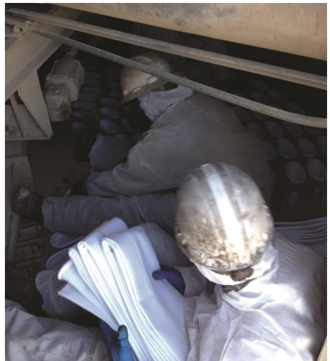
Replacing a baghouse with a cartridge dust collector improves worker safety by eliminating the dangerous confined-space entry required for bag filter changeouts.
